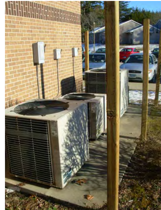
16. Exterior HVAC system condenser-compressor units
