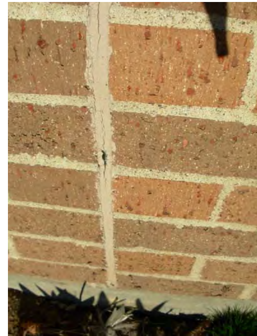
6. Drying and cracking of vertical control joints
