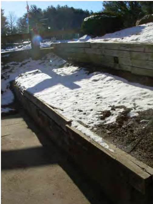
3. Deteriorating wood retaining walls to re-build Maple Courts II • Capital Needs Assessment • © On-Site Insight
