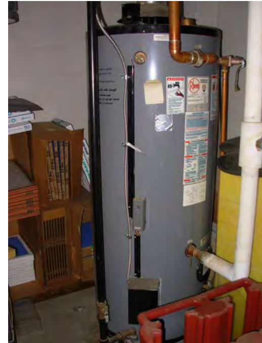
14. Larger DHW tank serving the kitchen facility
