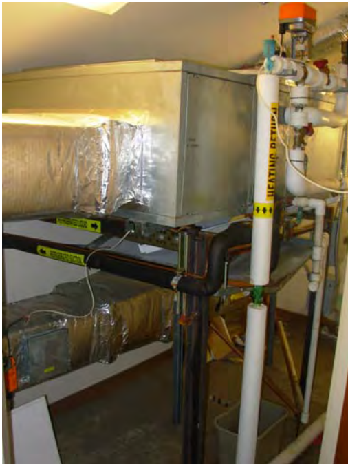
15. One of the HVAC system air handlers
