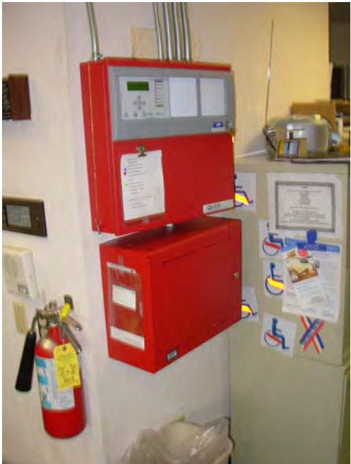
19. Fire detection system to be updated
